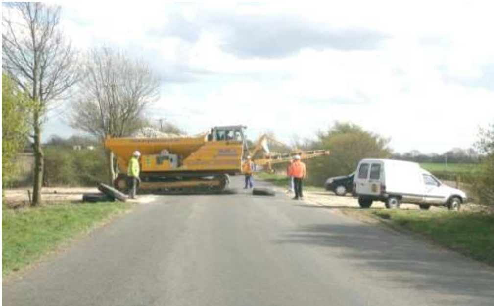
Figure 1: Typical Plant Crossing - Heavy plant crossing a road on a “haul route”.
